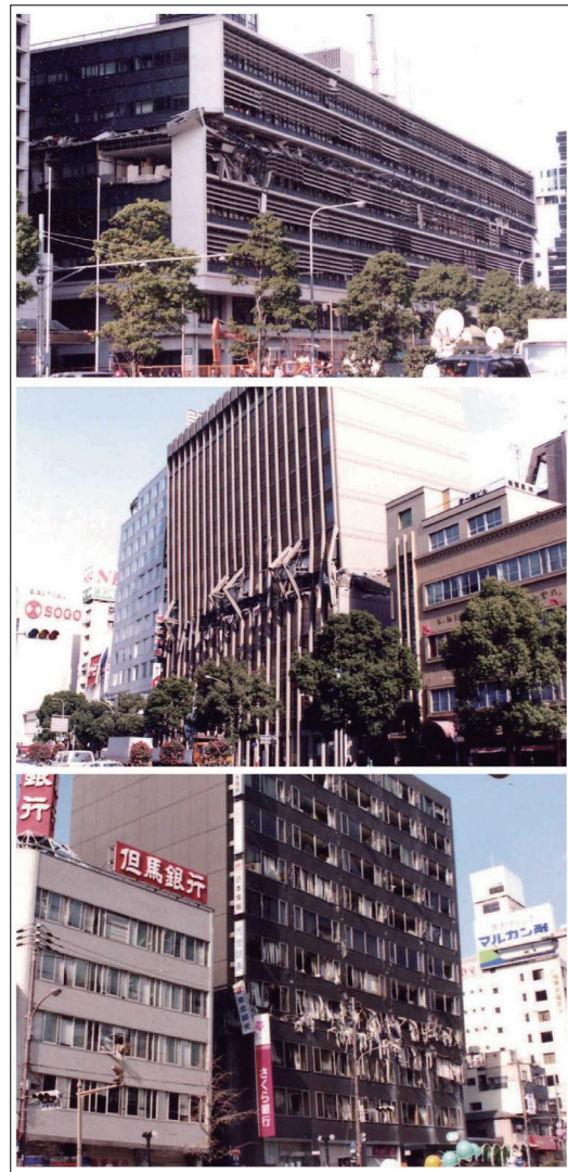
Figure 8 : Story collapse of Large Buildings. (Provided by Y. Sakai)
